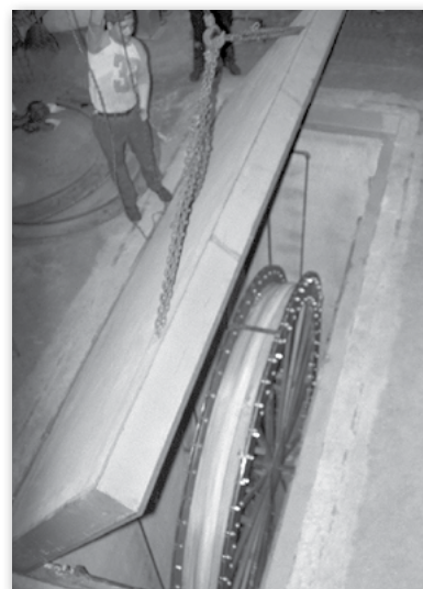
Raising of 10" concrete cover after completion of cure, prior to removal of product.
